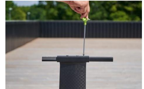
**2** Start with screwing the rear screw (above the thinnest part of the mast) then the central screw and only lastly the front screw. Tighten firmly and repeat several tightening efforts on the 3 screws.
